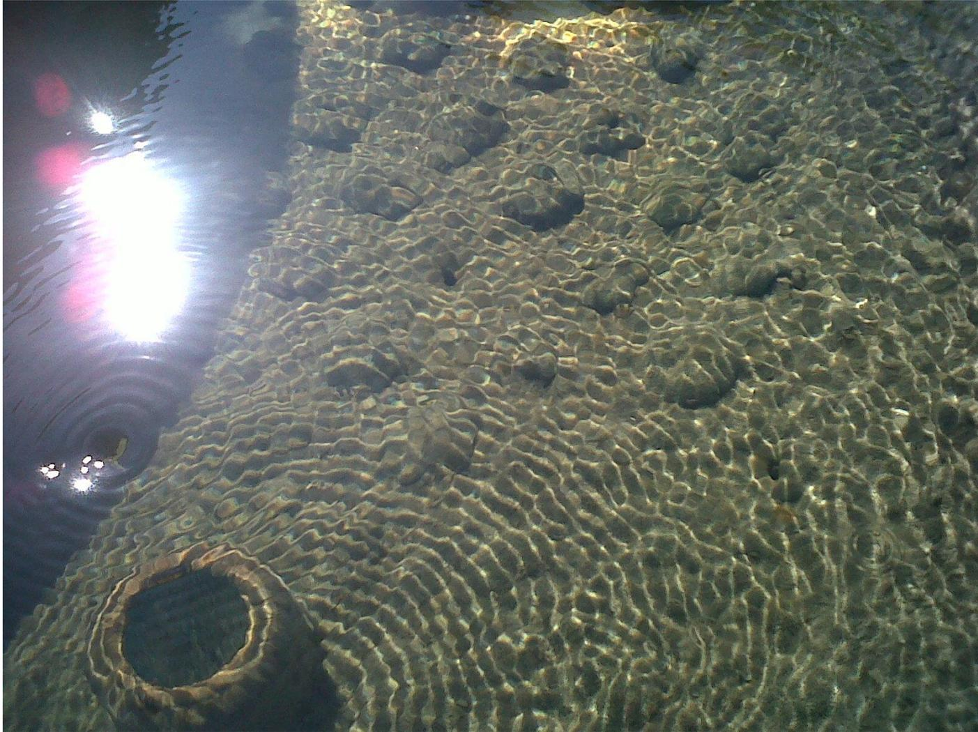
Algae deposited in hot water basins and water distribution holes become clogged
