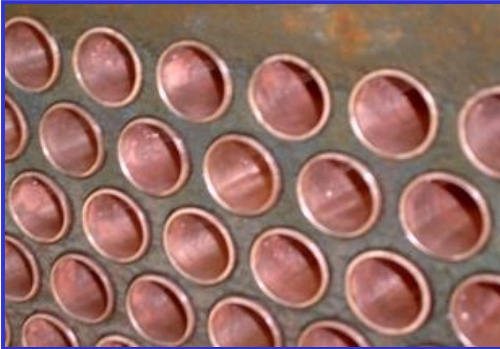
Condenser tubes after cleaned with the brush
