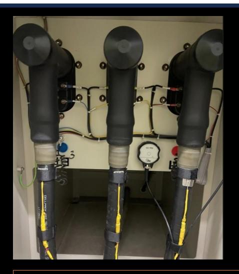
Vibration sensor and temperature sensor for panel
