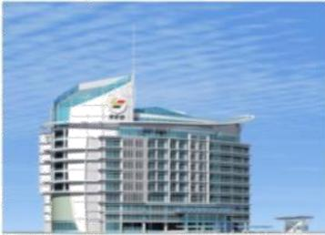
The building's main axis of orientation is parallel to the east-west axis and most of the windows are facing the north and south to reduce excessive heat gain.
