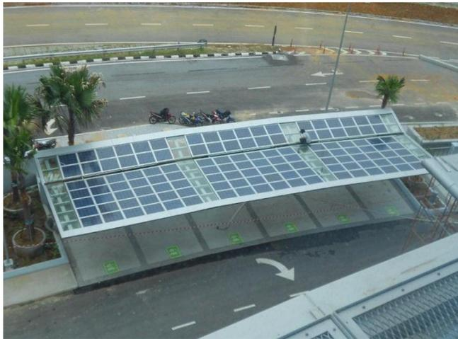
Building Integrated Photovoltaics Panels (BIPV)
