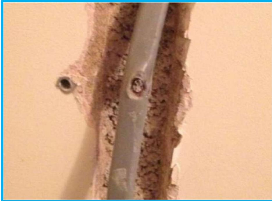
Wire damaged by drilling
