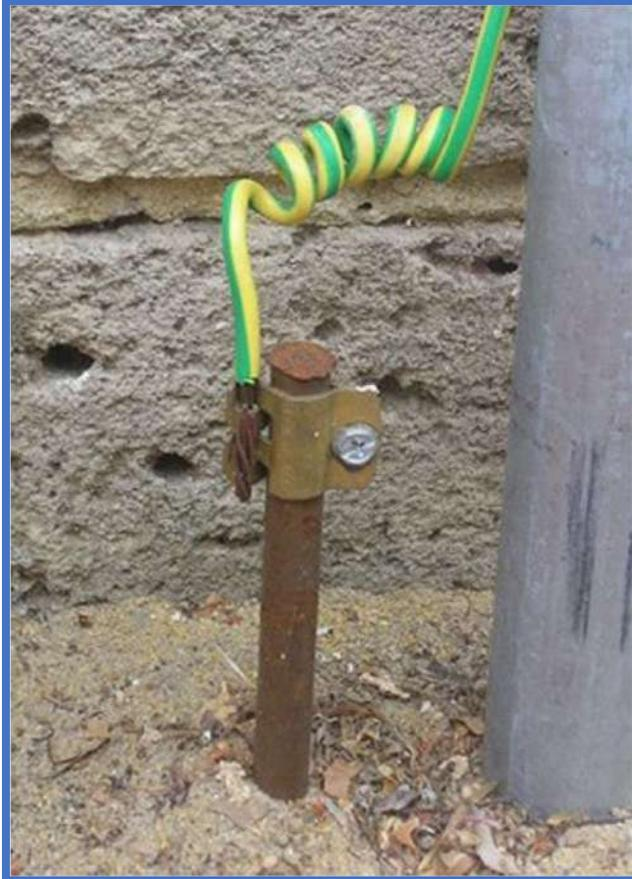
Earth Resistance Measurement is a direct measurement of the ability of the grounding system to dissipate current into the soil
