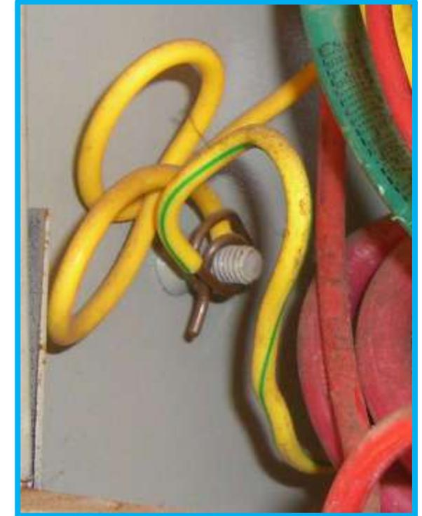
Every bad connection in the grounding system adds to earth resistance
