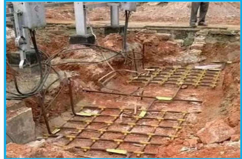
Choose the correct method to connect into the soil, based on measured resistivity of the soil
