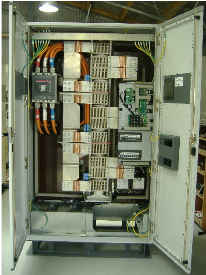
4000A Disconnect Switch
