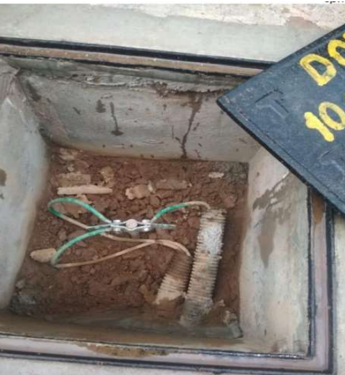
All the inverter Earthing risers are connected to the single earth electrodes.
