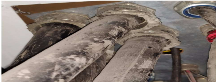
FIGURE-4: PE BAR EARTHING AT REMOTE POWER CABINET IS MISSING
