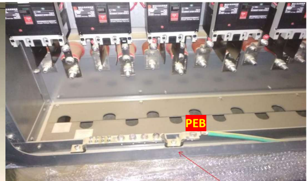
FE bus and PE bus is interconnected inside inverter.
