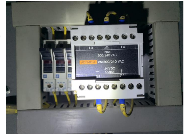
Power supply 24VDC for Trip unit: Generac AD 240 A VM Relay 200/240 VAC
