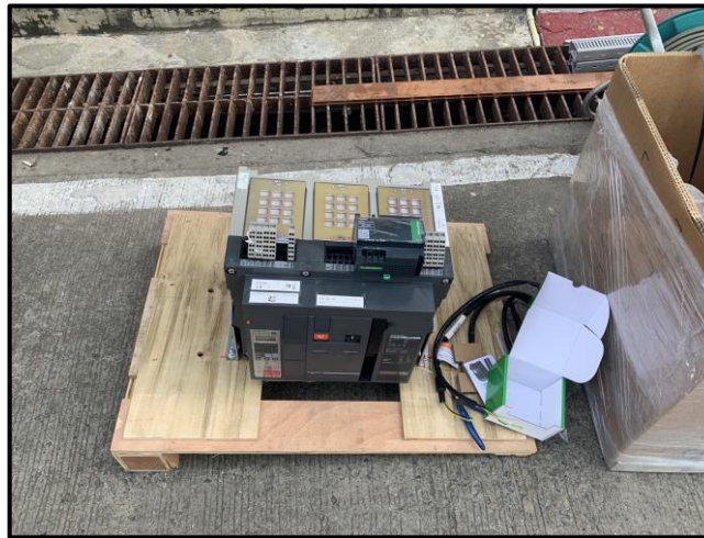
New ACB: manufacture Schneider model Masterpact NW16H1 1600 AT Fixed type Trip unit Micrologic 6.0 E
