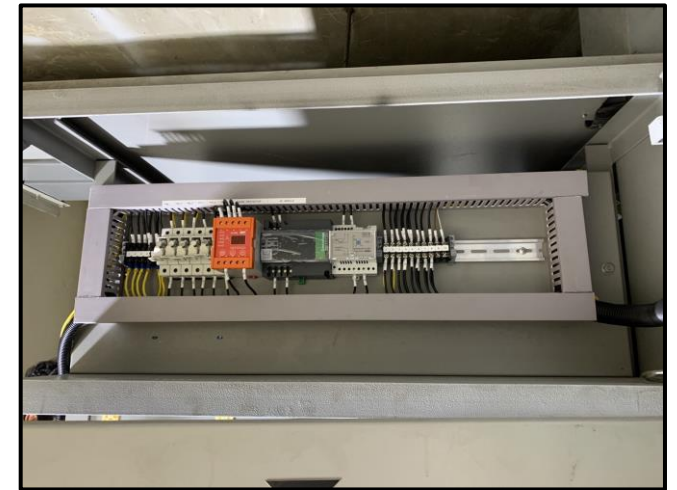
Additional : Phase Protection Model : W-PR3, UVR (under voltage release)
