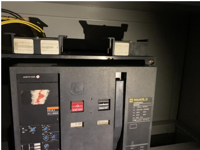
ACB: Square D master pact 16M H1, 1600AT, fixed type
