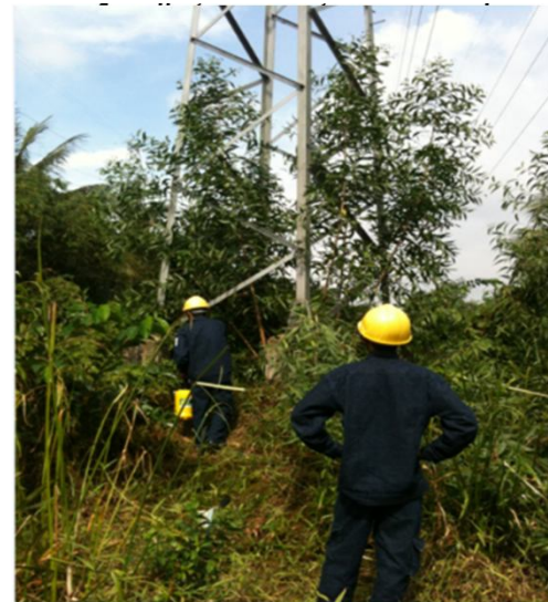
Regular site patrol and inspection
