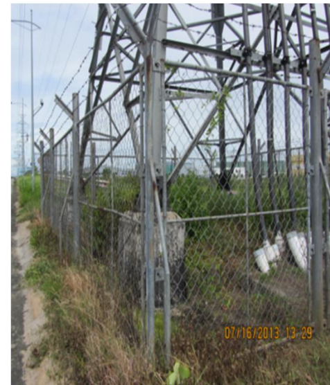
Installed extra fences to protect electric poles in high risk areas
