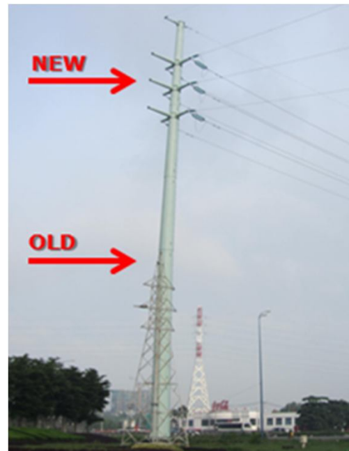
Upgraded height of existing electric poles to maintain a
