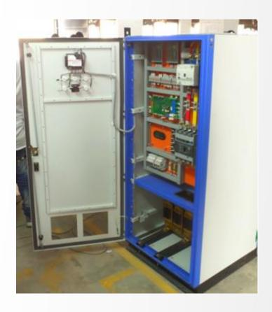
10,000A+ of Active Harmonic filters 7000+ Kvar of passive filters
