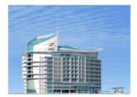
The building's main axis of orientation is parallel to the east-west axis and most of the windows are facing the north and south to reduce excessive heat gain.
