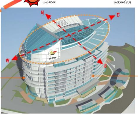
Generous glazed facades are lined along the north and south elevation. These facades are exposed to minimal direct sunlight and are featured with glazed curtain walls.
