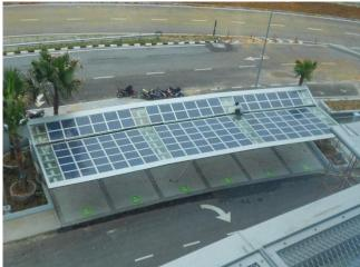
Building Integrated Photovoltaics Panels (BIPV)
