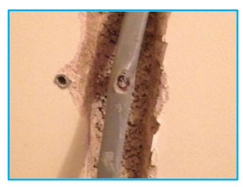
Wire damaged by drilling
