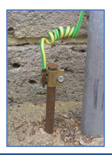
Earth Resistance Measurement is a direct measurement of the ability of the grounding system to dissipate current into the soil
