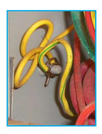
Every bad connection in the grounding system adds to earth resistance
