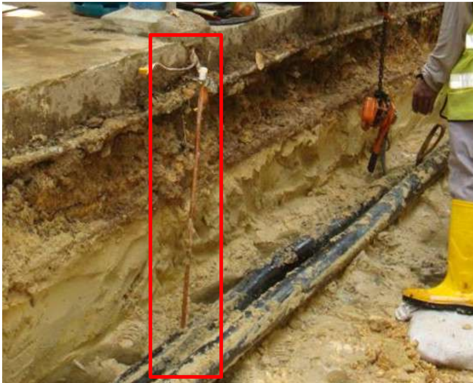
Earth Rod Sunk Into Transmission Cable
